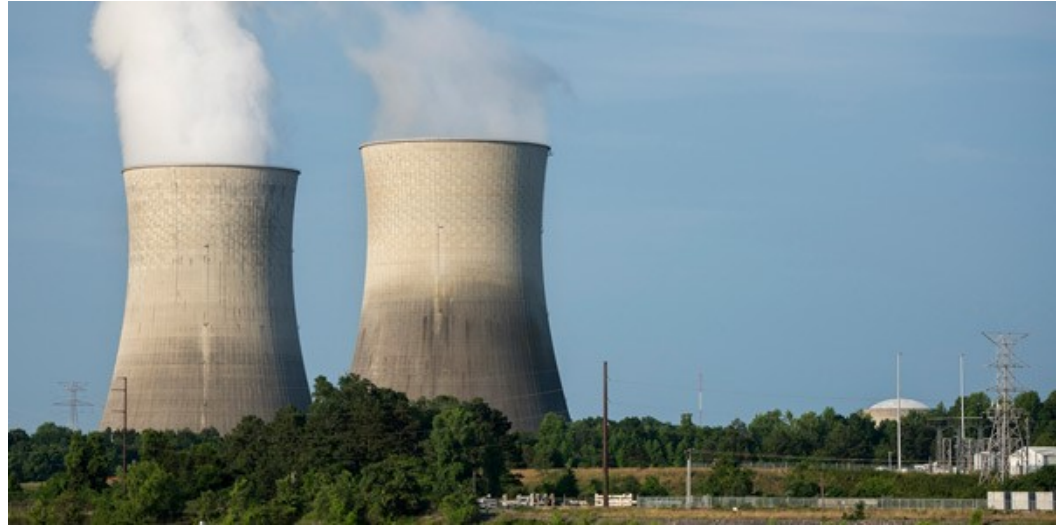
Watts Bar nuclear plant | TVA
